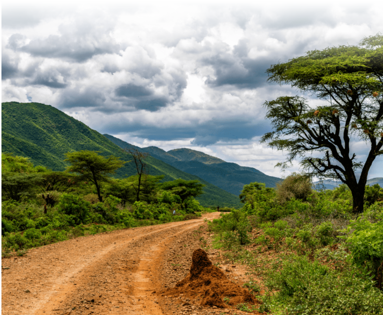
A County Government maintained road runs at the foot of the Tugen Hills
