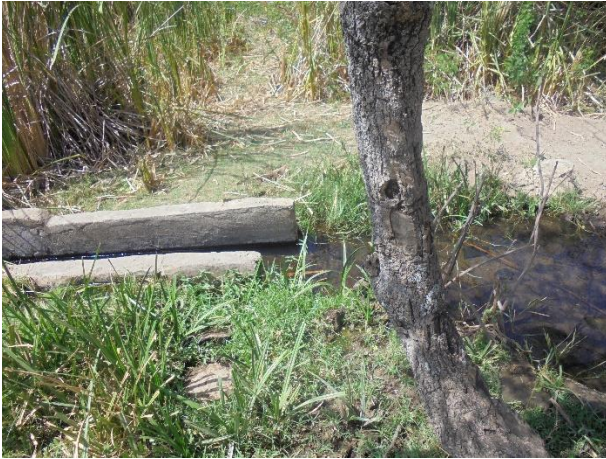
Lined canal for irrigation in Swamp water
