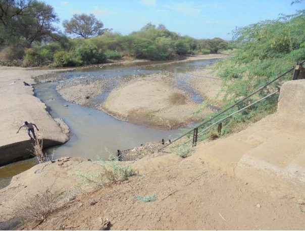
Perkerra irrigation scheme intake
