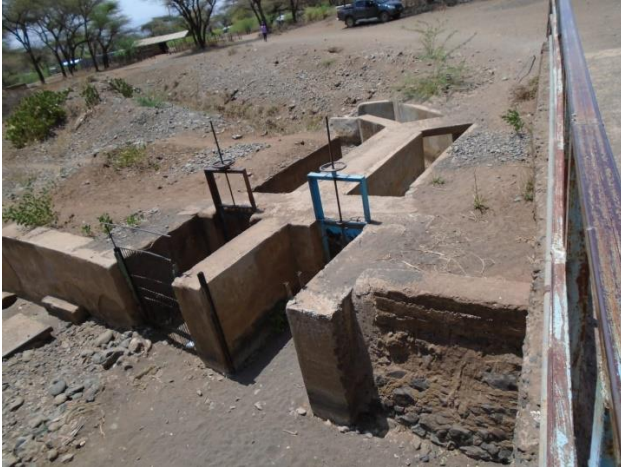
Sandai scheme water intake
